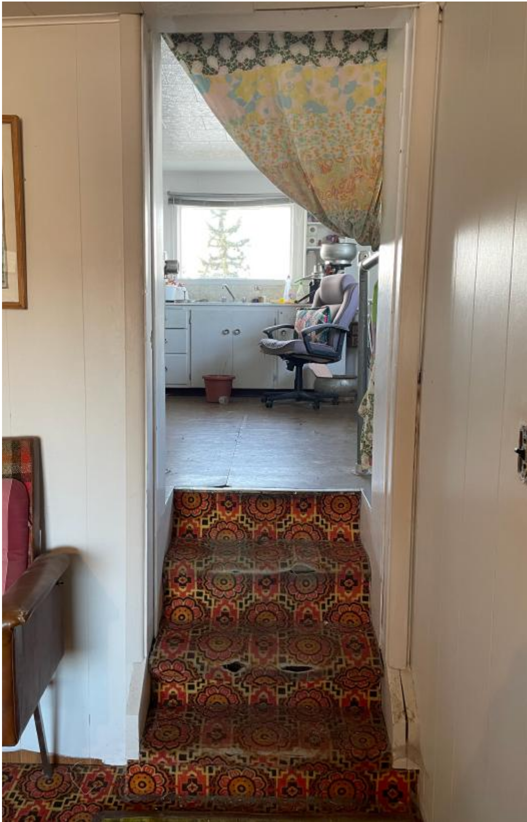
Figure 1 - Staircase between the living room and kitchen of the farmhouse. In this photo, the blanket covering the doorway is pulled to one side.
